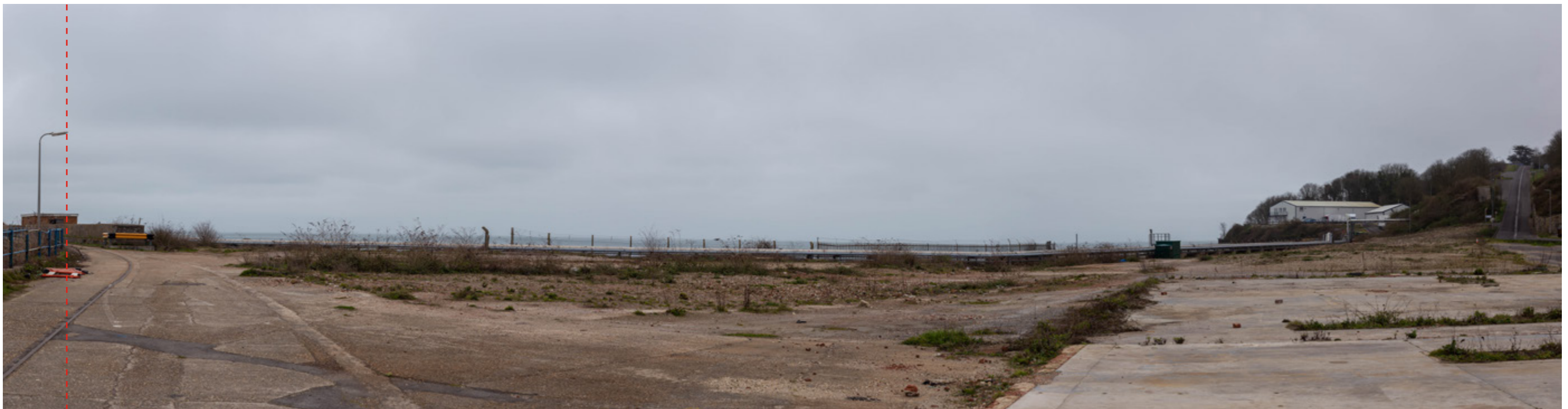
View along the upper level of the breakwater
