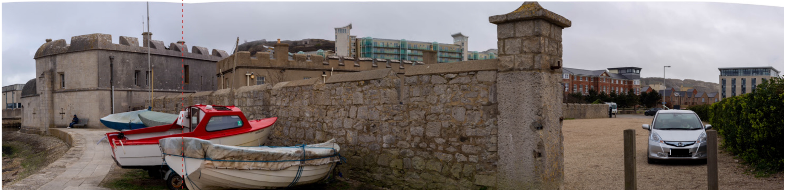
View along the shoreline
