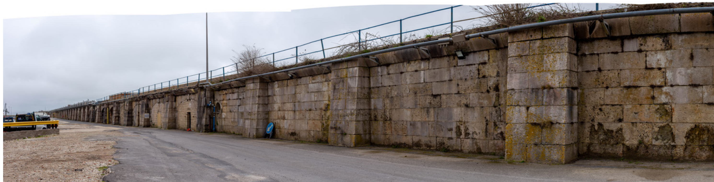
Two views along the lower level of the breakwater showing the coal storage casements
